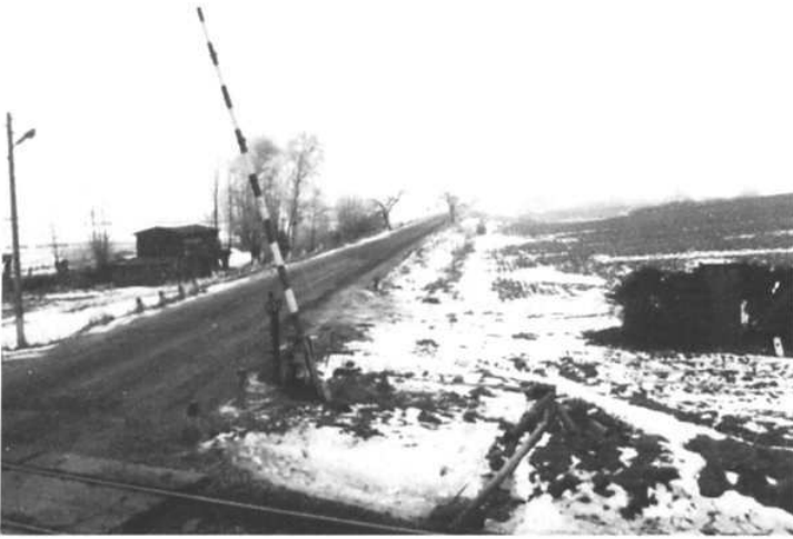
Photo 1: The railway crossing some months later.
